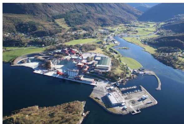
The olivine manufacturing plant at Åheim
