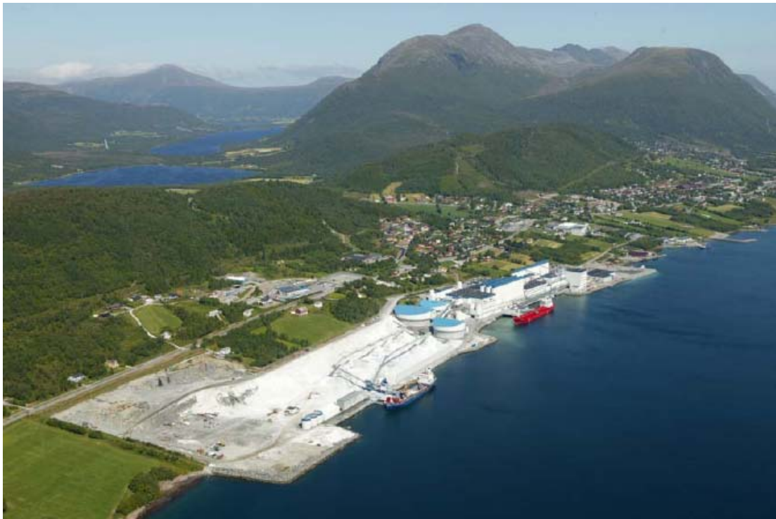
Hustadmarmor AS. Raw material storage and raw material ship nearest, processing plant and tank ship loading liquid marble in red.
